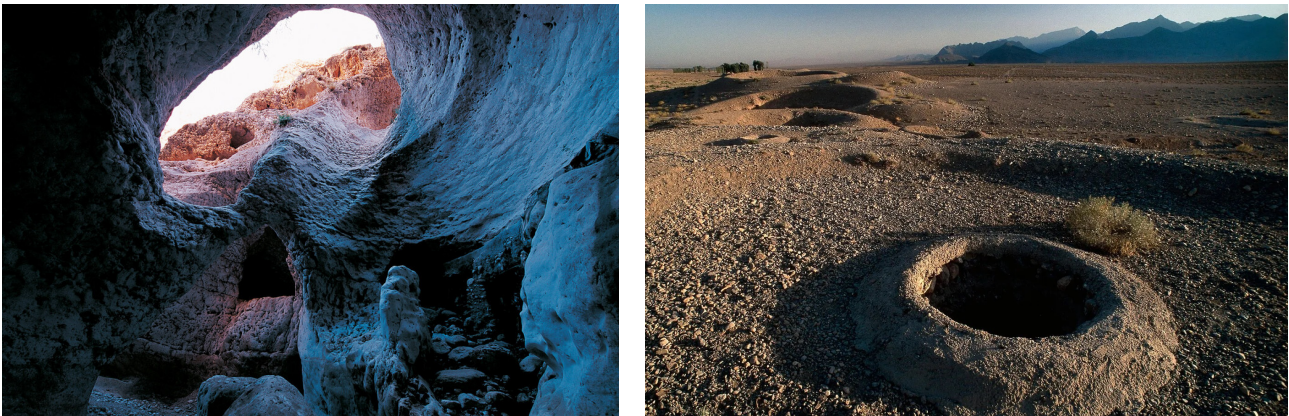
Image 20-21 Underground and surface manifestations of the Iranian qanat system used for water transportation and storage. In addition to providing water, qanats also help in cooling buildings and even preserving ice in some cases.
