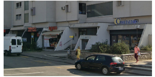
figure 10. - public base of a residential building in Podvežica
