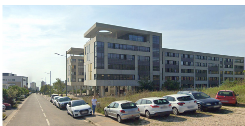
figure 41. - dormitory buildings with exclusive rooftop areas for informal interaction
