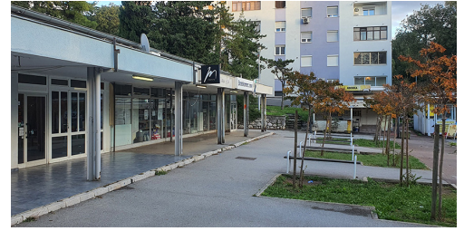
figure 8. - retail pavilion with a public space and surrounding improvised kiosks in Podvežica
